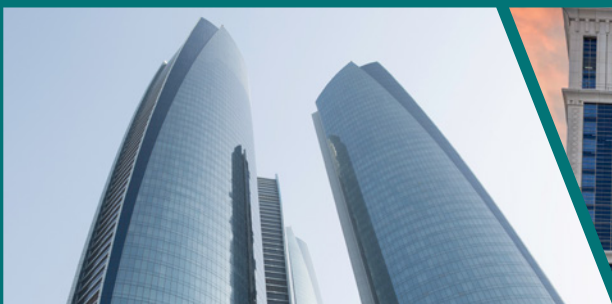
Etihad Towers, UAE (465,000m 2 )
